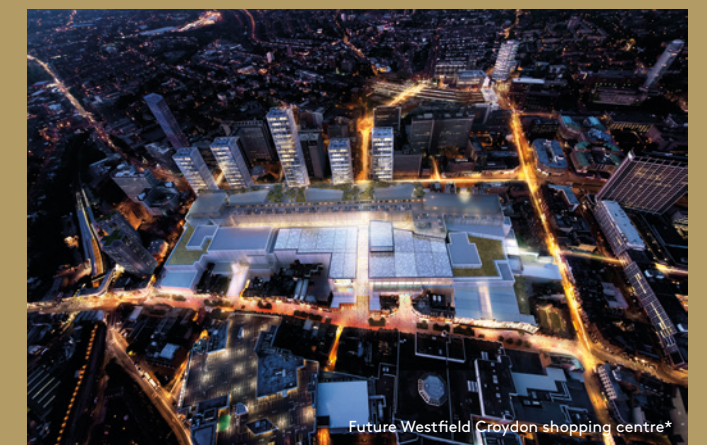
Future Westfield Croydon shopping centre*
